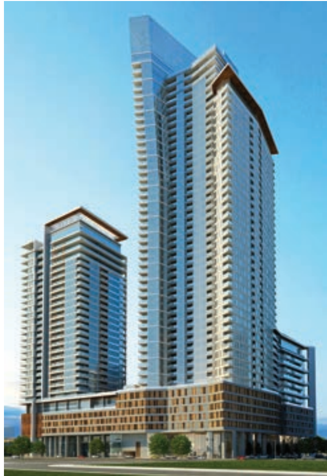
GILAN TOWERS BAKU, AZERBAIJAN
